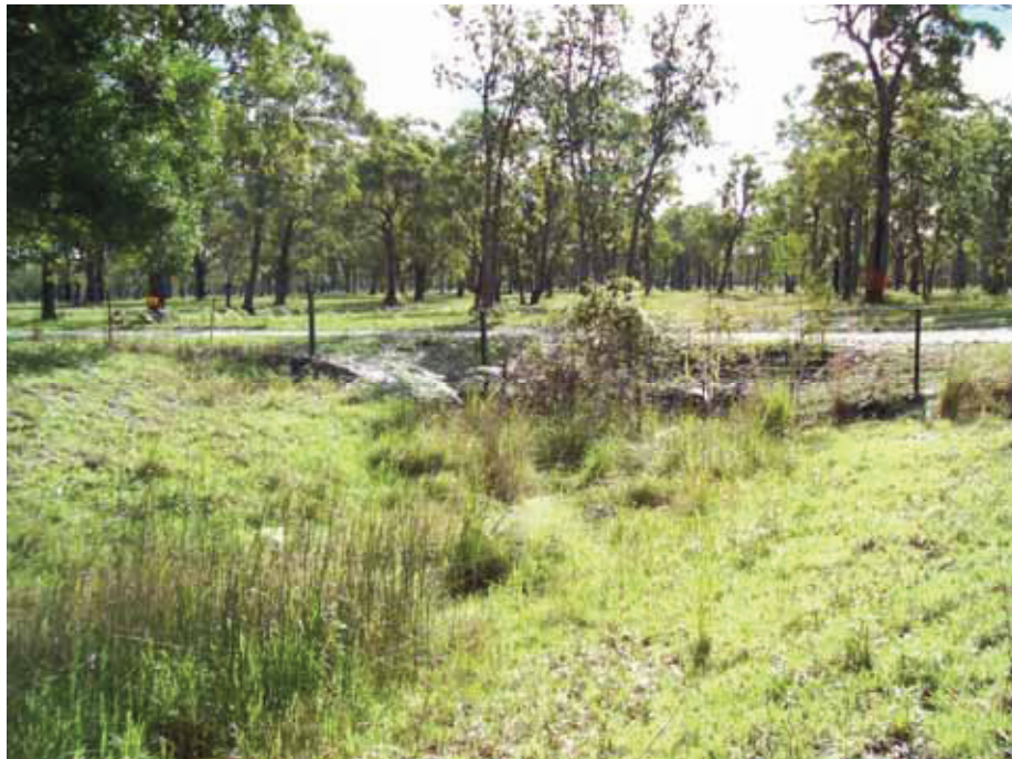
Plate 10 M2 drainage culvert from north east extent of M2.
